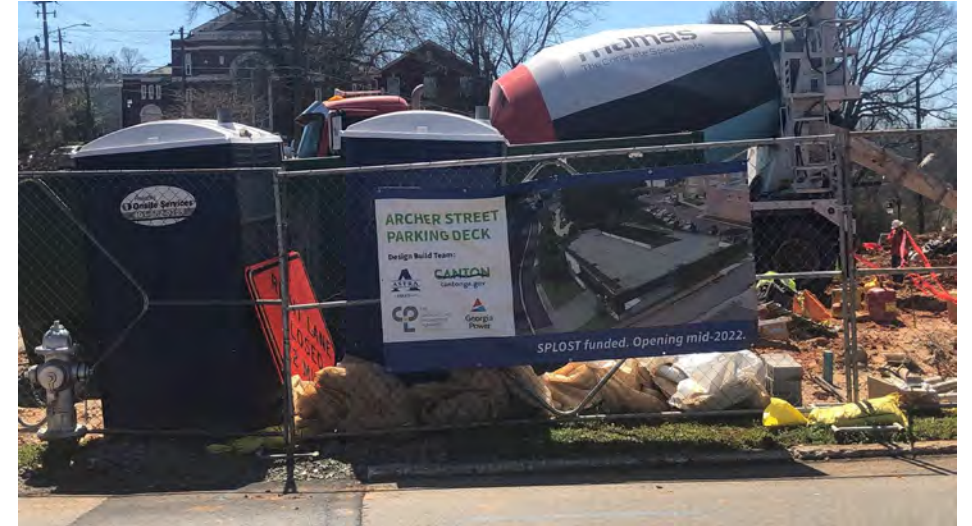
Construction Site of Parking Deck at Archer Street and Church Street
