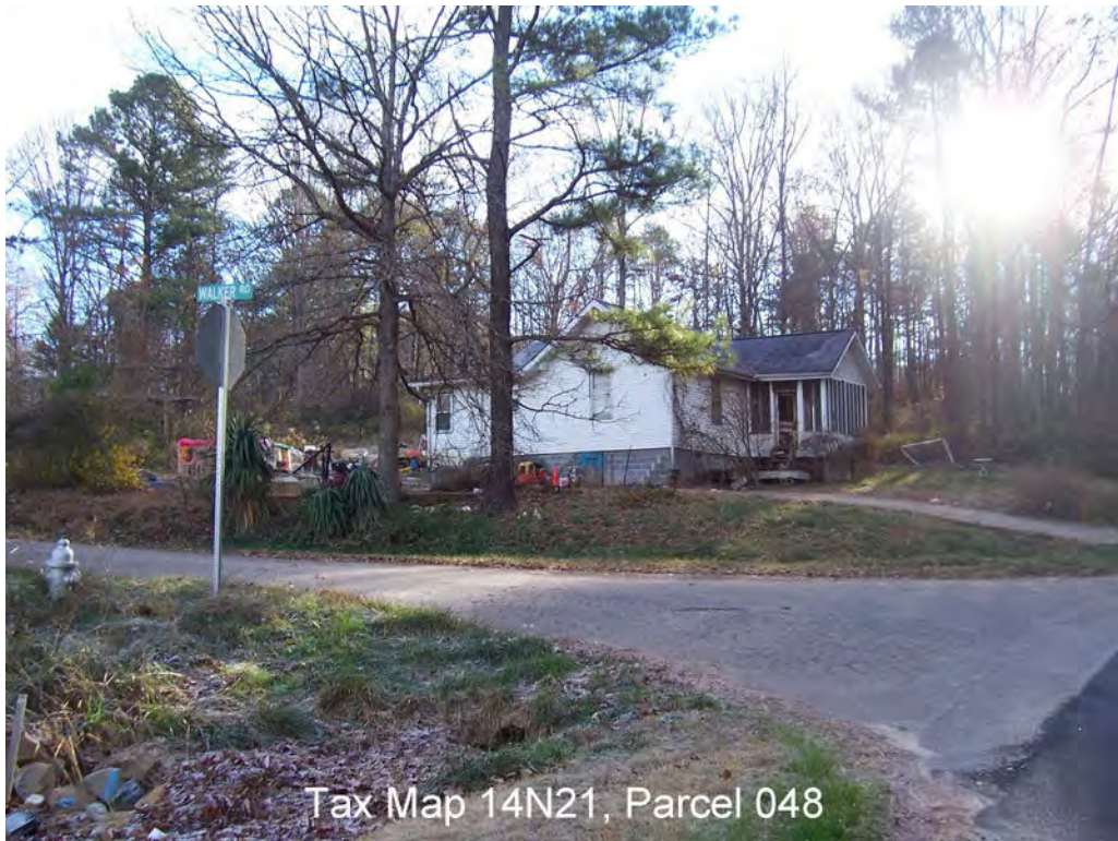
Picture 51—Distressed Residential Property
