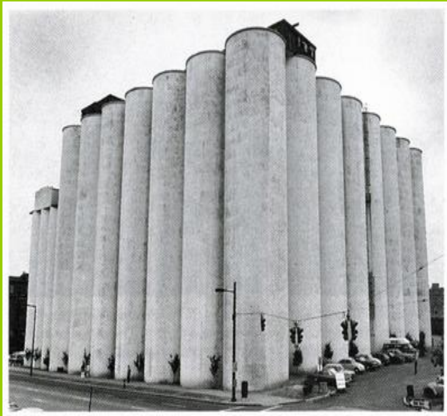
Quaker Oats Grain Elevators - Before
