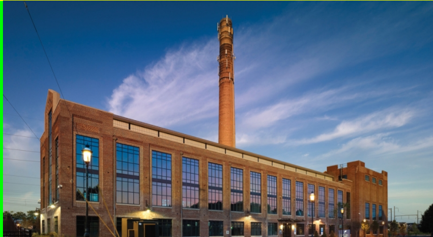
Boiler House Offices, Ambler, PA
