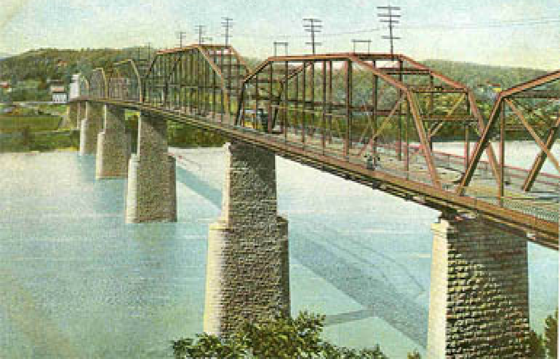
Hamilton County Bridge, over Tennessee River, Chattanooga, Tenn.
