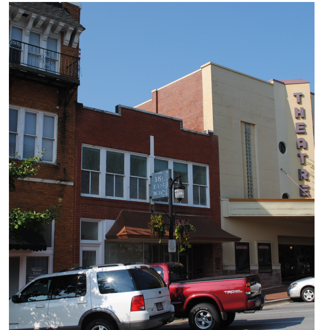
Commercial buildings within the historic district range from one to multiple stories in height.
