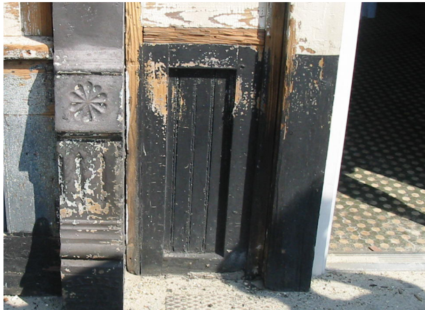
Original bulkhead materials should be treated with care and retained and repaired, rather than replaced.
