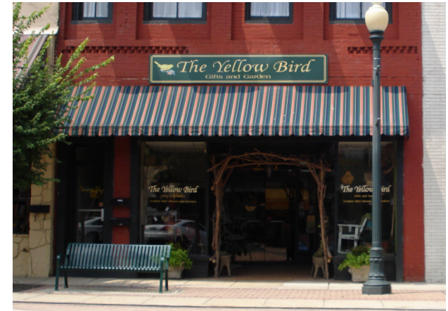
Awnings and canopies should match the width of the storefront and fit within the piers of the building.
