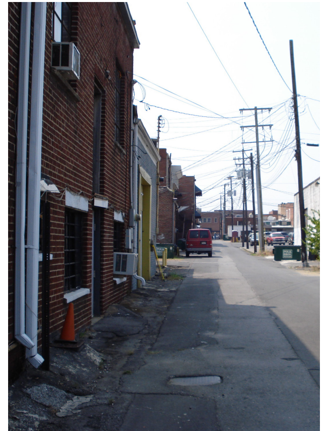
Alleys can provide a location for utilities that is hidden from most streets and sidewalks.
