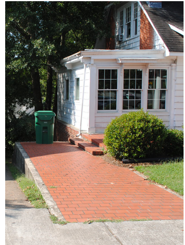
Brick, stone and concrete are appropriate materials for driveways and walkways. Original materials should be maintained and preserved.
