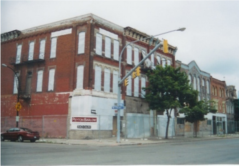
A building that is properly stabilized can be secured and preserved until a viable new use for the building can be found.
