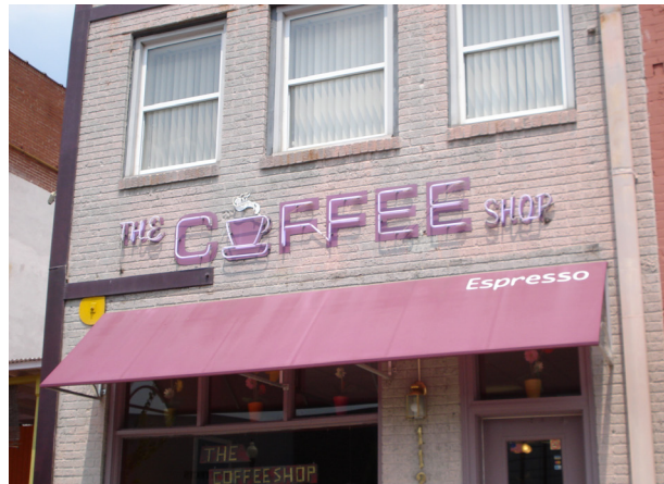
Awnings can be placed in front of transom windows to provide shade from excessive sunlight. This application is primarily for south facing storefronts that receive abundant sunlight during the day.
