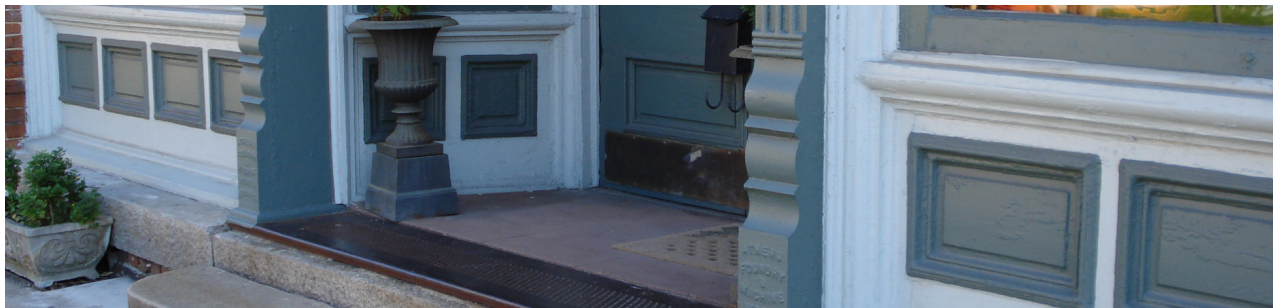
Panels and other architectural ornamentation is commonly used with bulkheads to create visual interest around the storefront.
