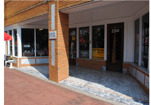
Storefronts can be flush with the street or recessed to provide shade or cover from the elements.
