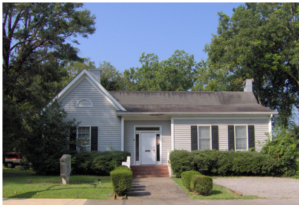
Walkways can be used to highlight or accentuate the entrance to a building.
