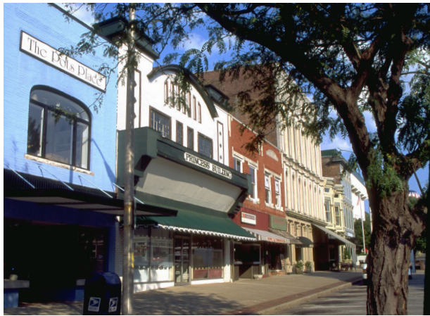
Balconies added to buildings should not obscure architectural features, such as windows or sign bands.
