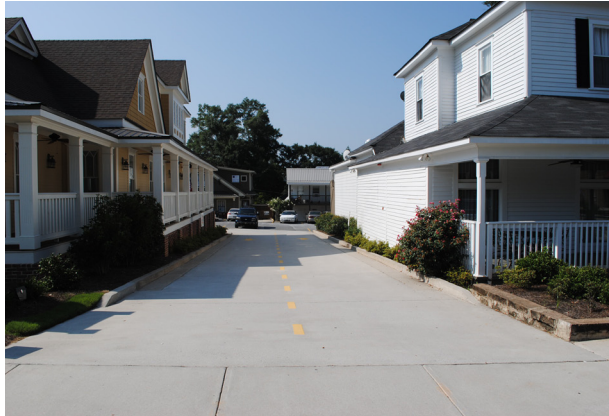
Shared driveways help reduce the number of curb cuts and the amount of impervious surfaces on a property.
