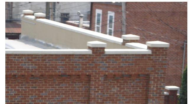
Contemporary cornices commonly include simple construction with metal, stone and/or masonry treatments.
