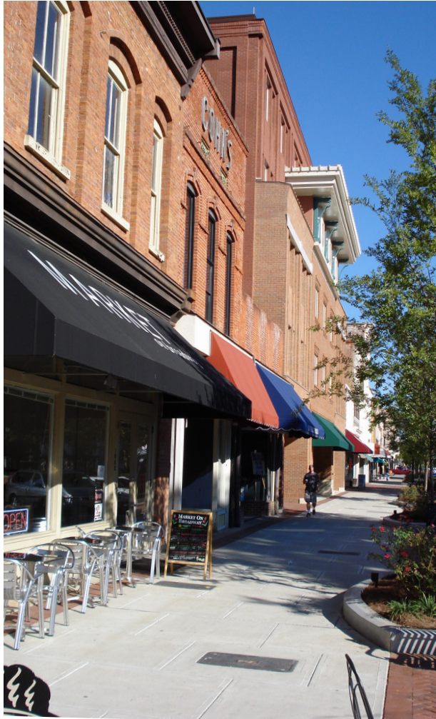
These storefronts vary in configuration along the street but they are all inviting to the pedestrian with transparent glass display windows and doors.
