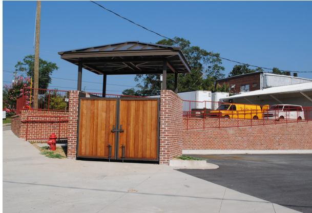
Utilities that require regular service, such as dumpsters, should be located for convenient access and screened with appropriate walls, fences, doors and/or landscaping.
