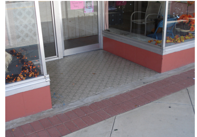
Contemporary bulkheads commonly use a single material for the base of the bulkhead with display windows set flush with the top of the bulkhead.
