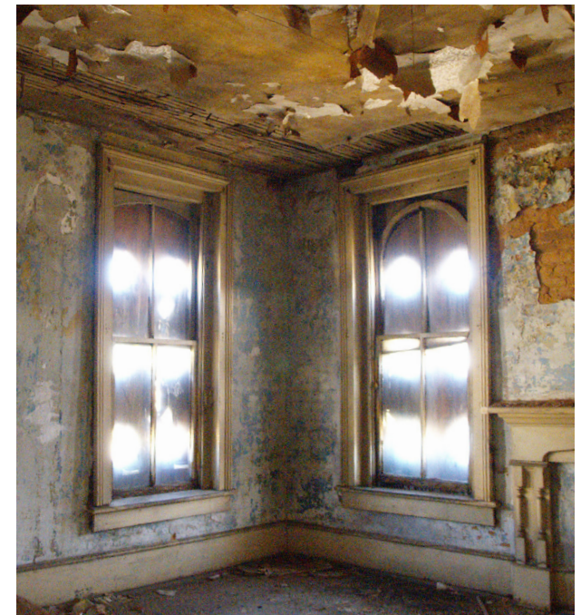
Original window materials should be retained and repaired, rather than replaced.
