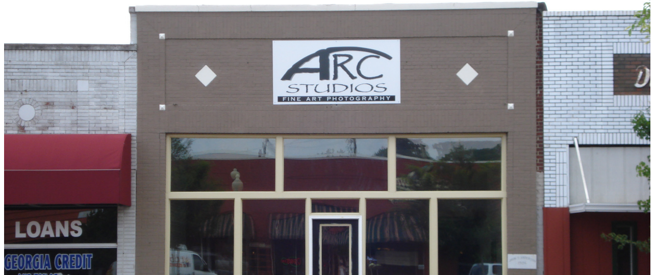
Transom windows are placed above display windows or entry doors to allow natural light in to the interior of a building.
