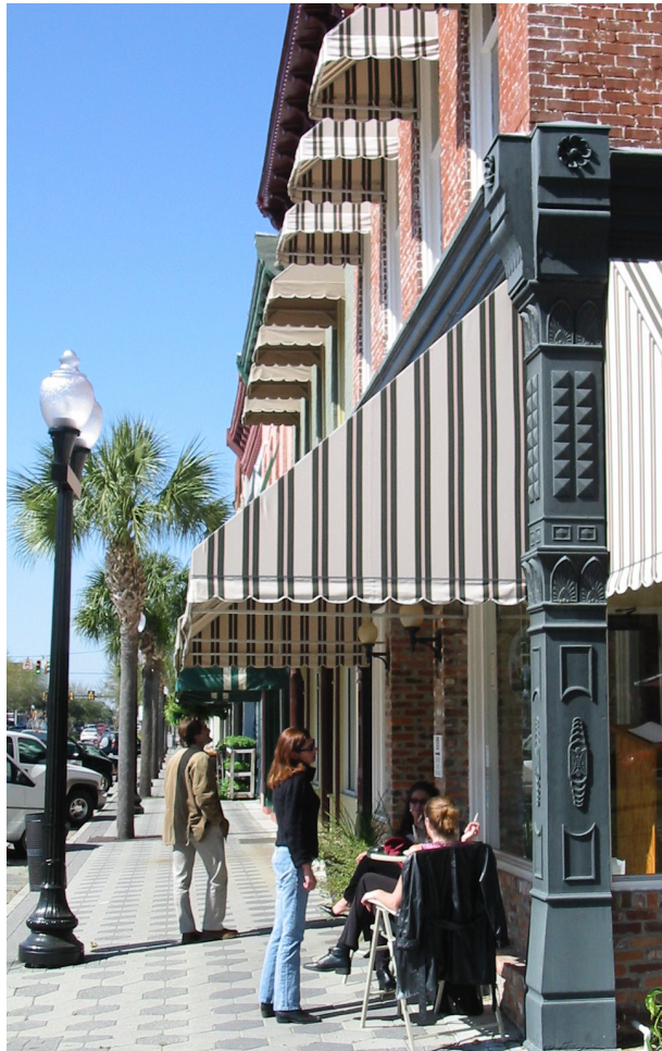
Awnings should project over the sidewalk to provide shade and cover from the elements for pedestrians or sidewalk diners.
