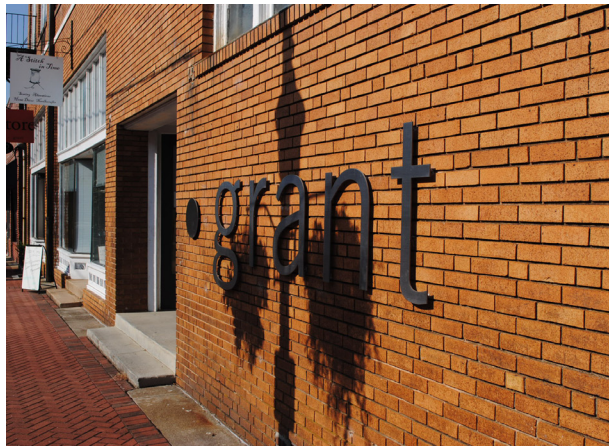
Metal or wood are appropriate sign materials for projecting and wall mounted signs.
