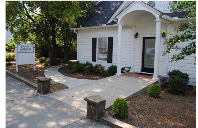
Walkways should enhance pedestrian access to buildings from the street or parking areas.
