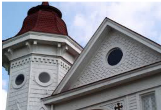
High-style Queen Anne Victorian, vernacular Victoria era farmhouses, and Folk Victorian gabled “L” cottages have a change of pattern and/or material with each level. One-story houses will have this treatment in the gable.
