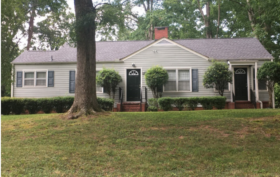
1260 East Main Street is a local example with elements of the Minimal Traditional style.
