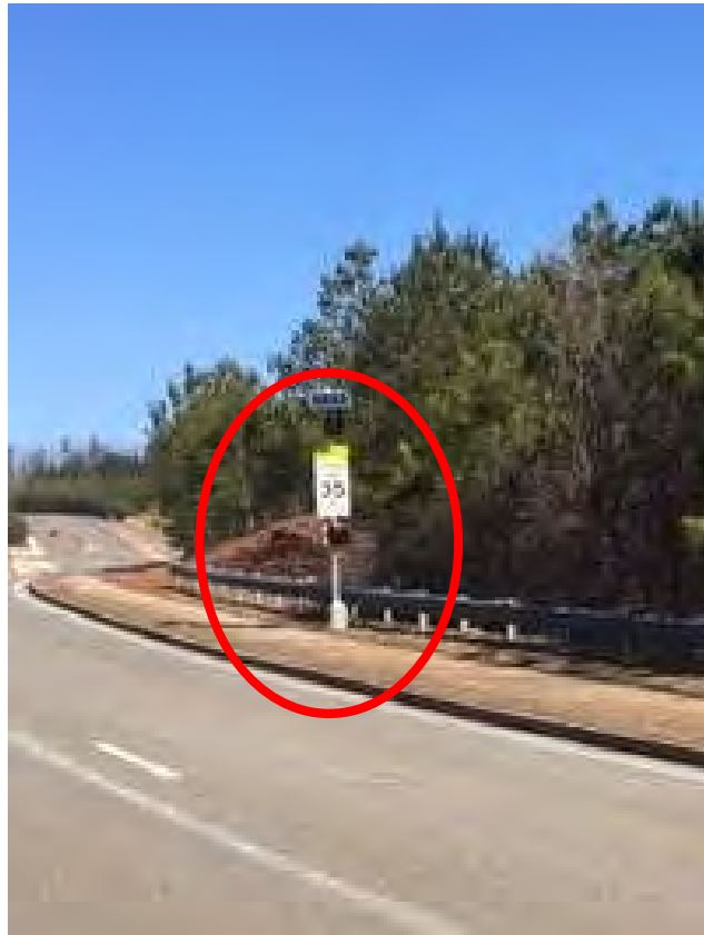
Figure 5. School Zone (Symbol) sign (S5-1) on Reservoir Drive Northbound
