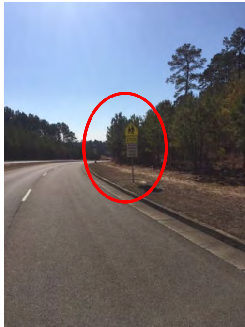
Figure 7. School Zone (Symbol) sign (S1-1, S4-3P, R2-10) on Reservoir Drive Southbound
